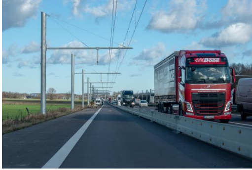
Figure 1: Construction of the overhead power line on the autobahn A1
